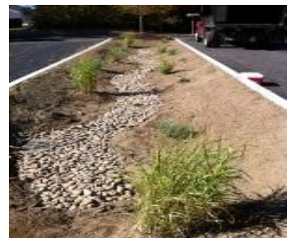
Bioretention system in Stratham constructed under the Biopalooza grant.
